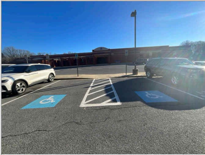
OVERVIEW OF ACCESSIBLE PARKING AREA
