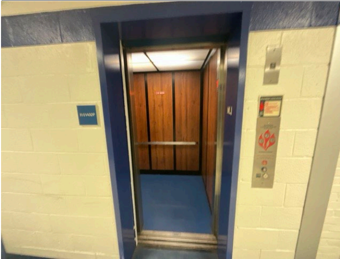
13 - ELEVATOR CAB FINISHES
